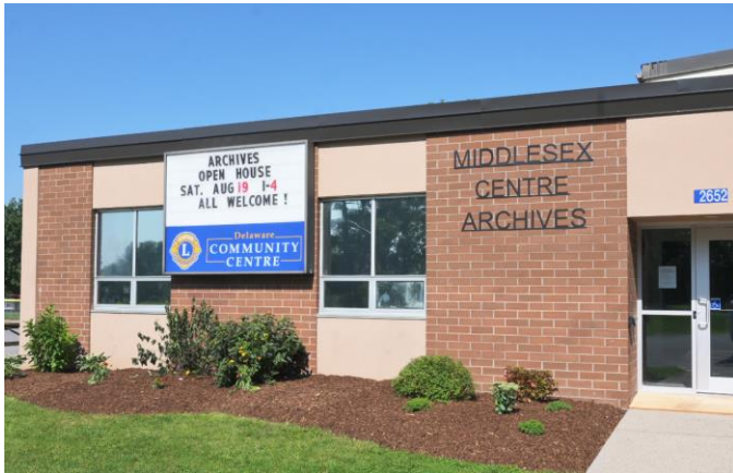
New Gardens and new handicap door entrance ( Thank you Middlesex Centre )
